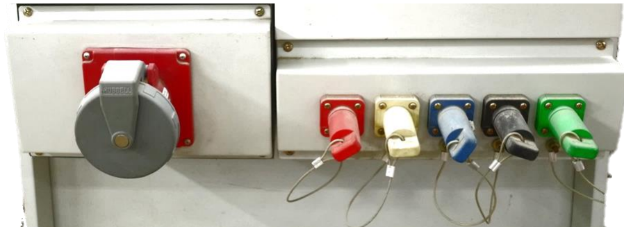
Figure 2.4 - Additional Power Supply
